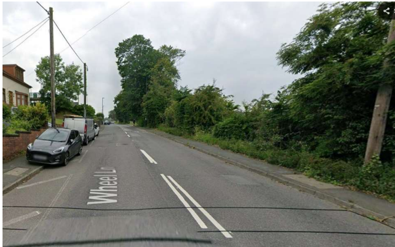
Wheel Lane Footways Narrow and Obstructed - Google
