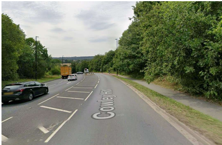
Cowley Hill Overgrown Footway - Google
